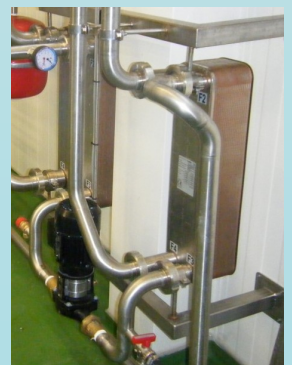
Heating with heat exchanger
